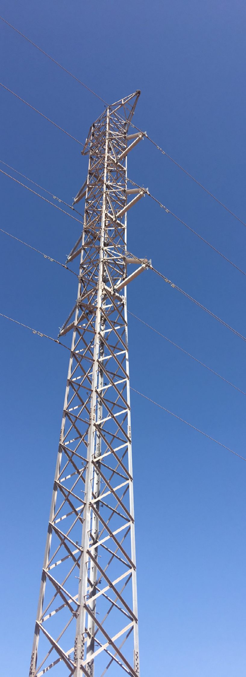
Bonomi's braced insulated cantilevers on some trellis in Fuerteventura, Spain
